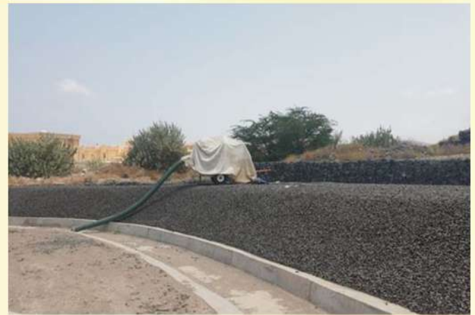
storm protection dam
