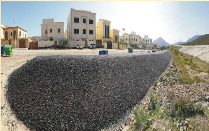
Slope reinforcement in Khorfakkan city, Al Mousallah project Sharjah (MOID)
